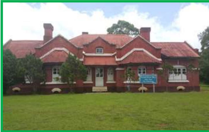
Figure 4: Hundred Years Aged-old Building
